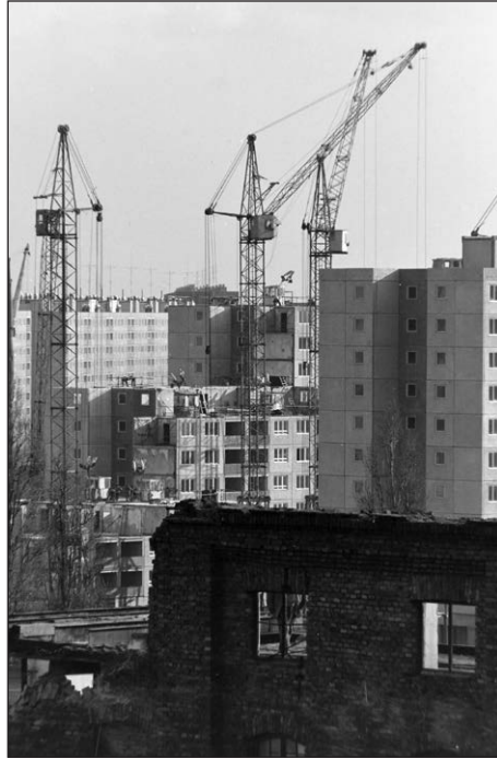
Figure 30. Construction of the housing estate in Óbuda, 1974 (Fortepan, 198870, Zoltán Szalay)
